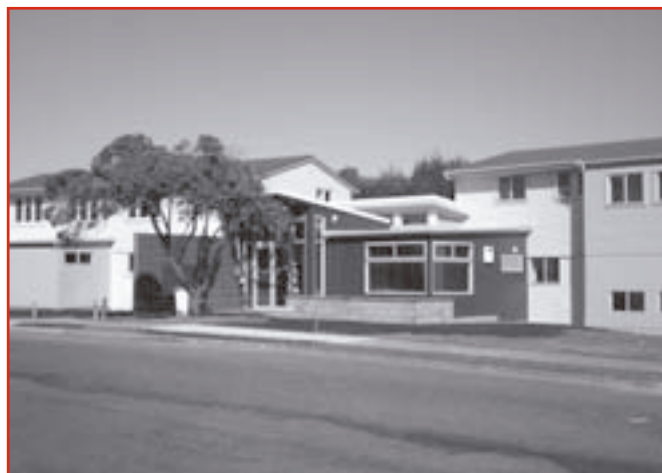
The Aoga Amata Porirua EFKS new facilities.
